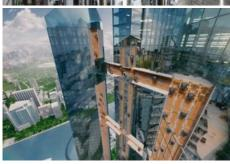
The MULTI revolution changes the way people move inside buildings, providing completely new perspectives for architects, real estate owners and passengers. By employing linear motors for each cabin, no ropes are needed at all - MULTI moves move vertically as well as horizontally. Editorial use of this picture is free of charge. Please quote the source: "obs/thyssenkrupp elevator AG"
