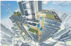
ThyssenKrupp's MULTI consists of various cabs per shaft and enables vertical and horizontal movement. Further text via OTS and www.presseportal.de/pm/113002 / Use of picture is free of charge. Please quote:: "obs/ThyssenKrupp Elevator AG"
