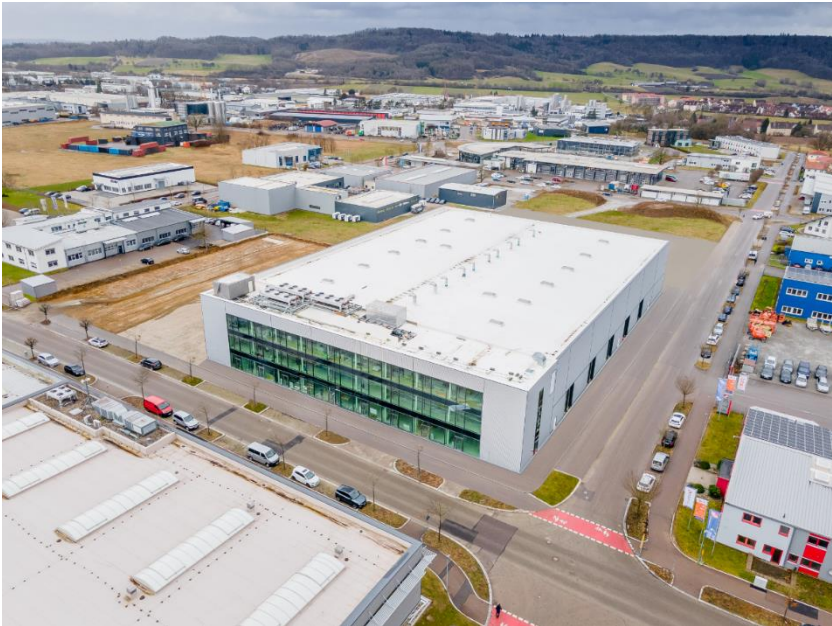
The opening of the new CSPE Center II (center) has increased Optima Pharma's production area in Schwaebisch Hall's Solpark business park by an additional 4,000 square meters. (Source: Optima)
