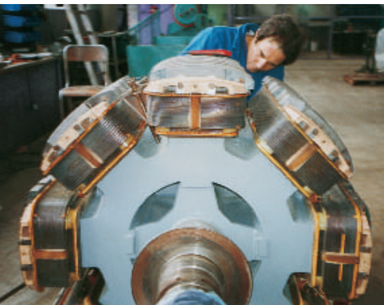
Added service value: with the acquisition of the French service provider EITB, we have strengthened our know-how in the repair and maintenance of electric motors.
