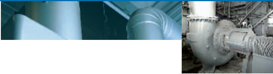
For a cleaner environment: large process pumps transport lime milk used for flue gas desulphurization in power stations.
