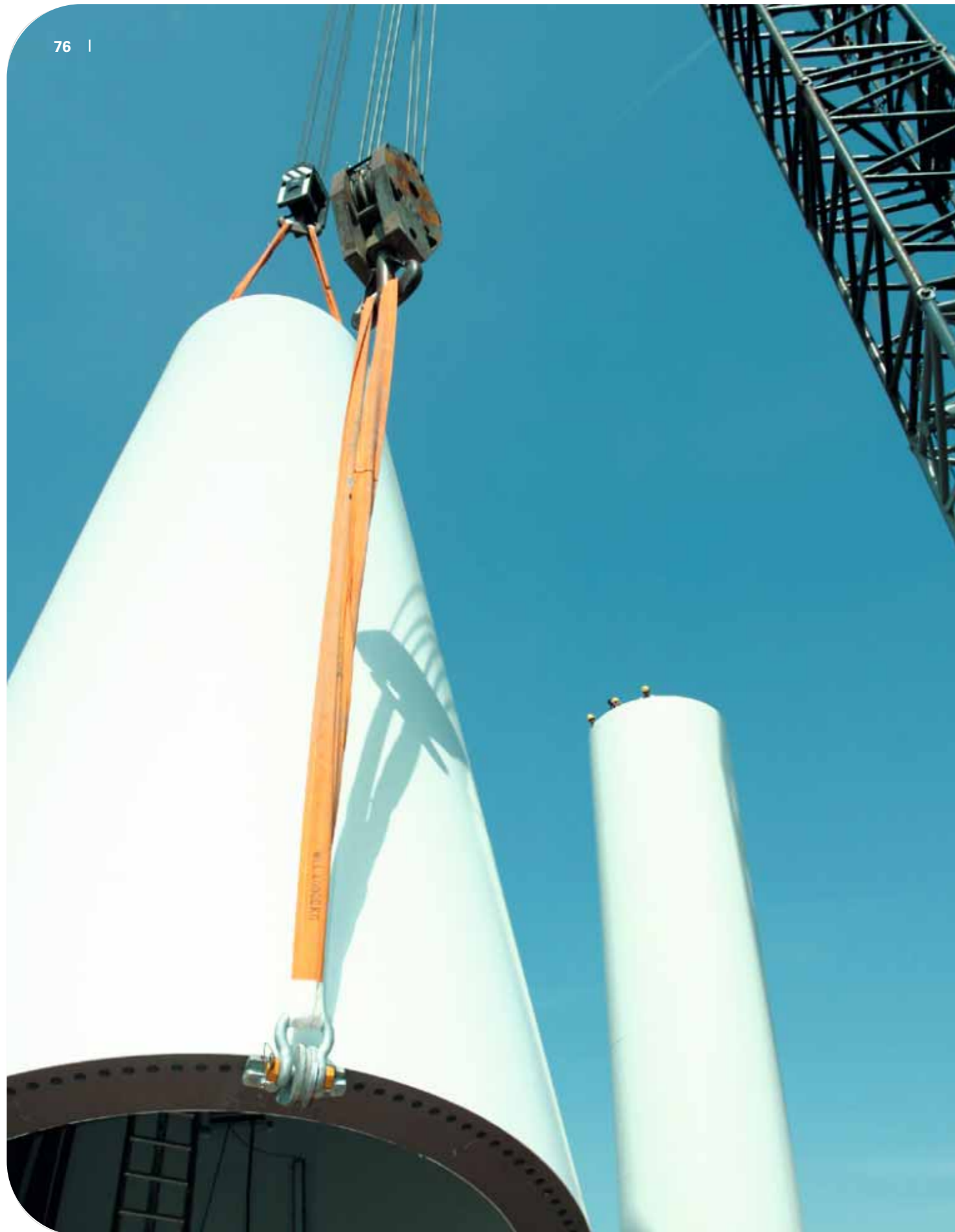
1 Tower segments being assembled | staff awaiting the next segment.
