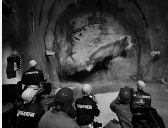
↑ Breakthrough in Switzerland on Friday for the world's longest tunnel. On October 15, 2010, at 2.17 p. m., 800 meters below ground, the tunnel drilling machine "Sissi" cut through the last remaining rock.
