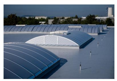
The LAMILUX Continuous Rooflight B is optimally suited for large-area illumination of halls with daylight.
