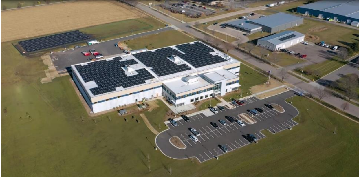
Image 1: Rooftop solar panels are just one of the eco-friendly features of GEA's new fabrication, repair, logistics and training facility in Janesville, Wisconsin (USA). Source: GEA
