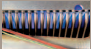
Gas boiler in operation
