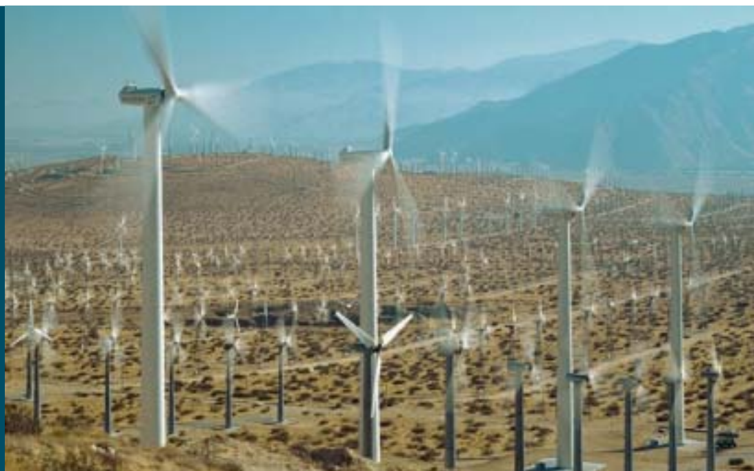
Endless energy from wind: wind farm in California.
