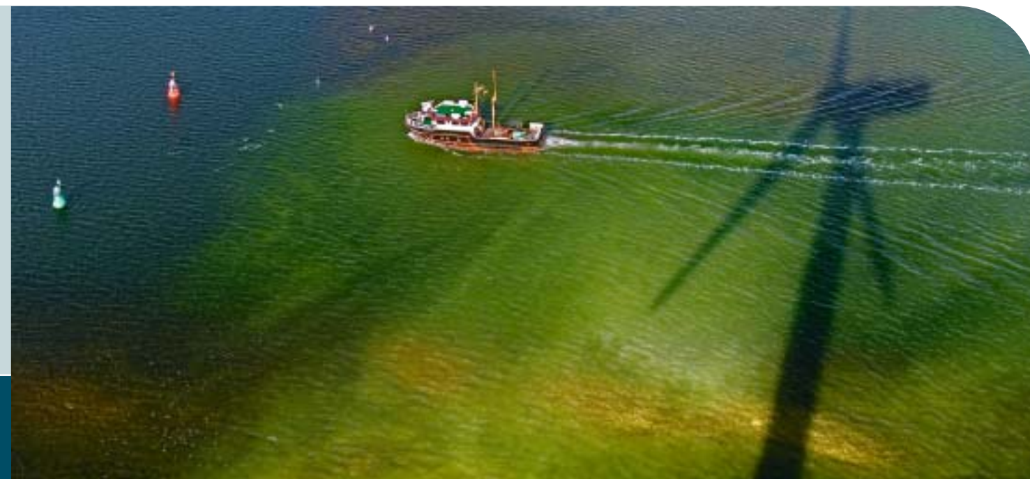
N90 Offshore – Main pillar in the water.
