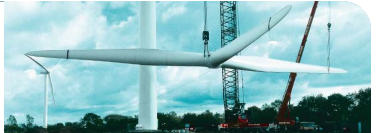
Installation times shortened due to rotor assembly in one step.
