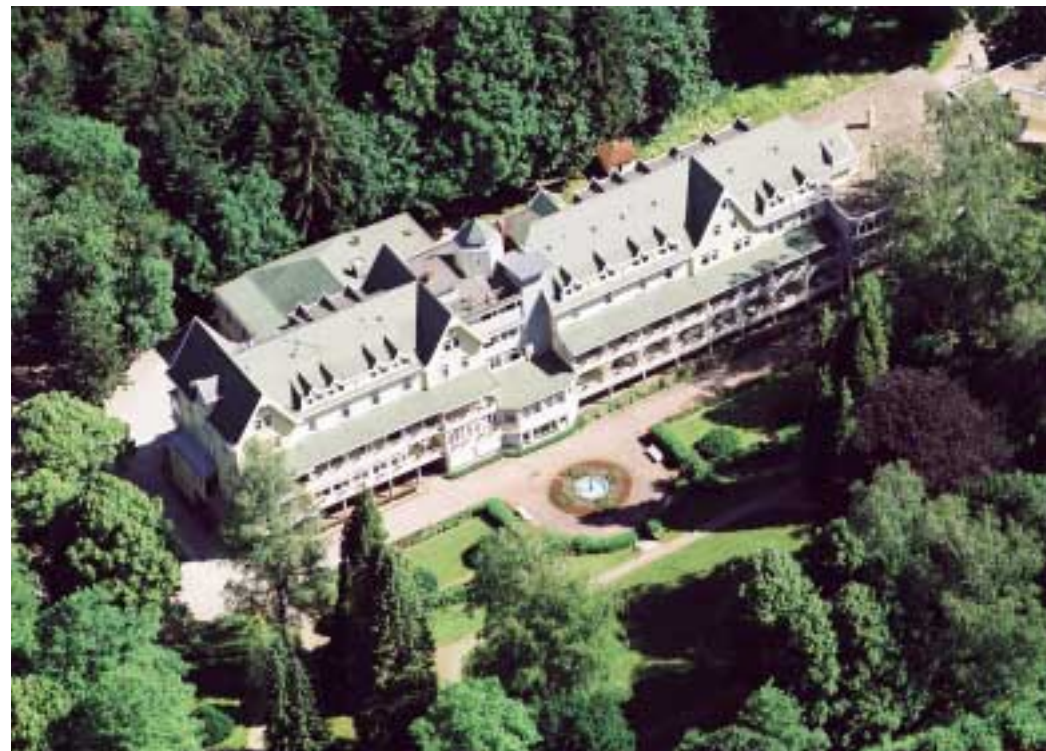
Schömberg psychosomatic clinic. The nursing clinic concept is being integrated here in future too in response to the changes on the health care market.
