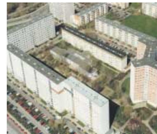
756 residential units in three blocks of flats: assisted living in Halle (Saxony-Anhalt).
