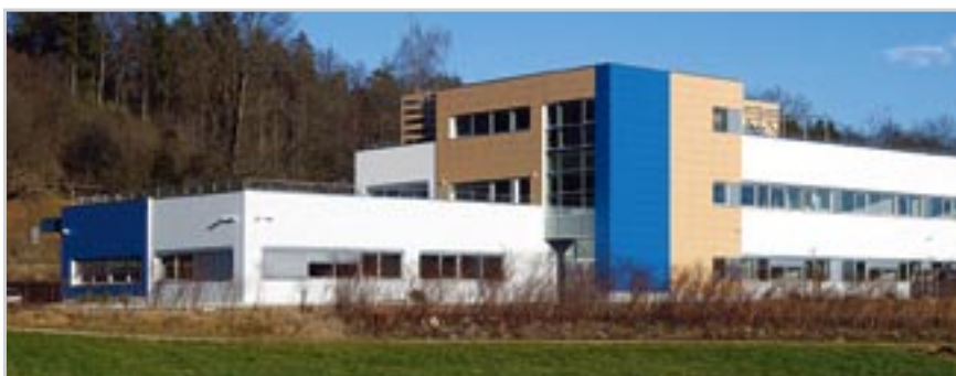
The new office and production complex for LPKF Laser & Elektronika d.o.o. in Naklo, Slovenia.
