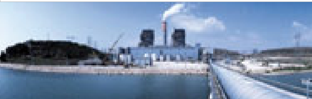
The Iskenderun Bay coal-fired power plant in Turkey is equipped with KSB boiler recirculation pumps.
