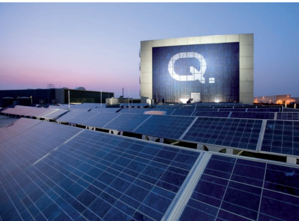
Solar-modules on the roof of Q-Cells in Thalheim
