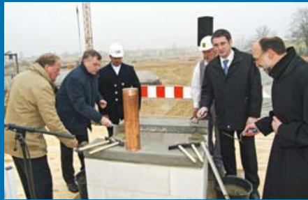
Laying foundations for new production facility
