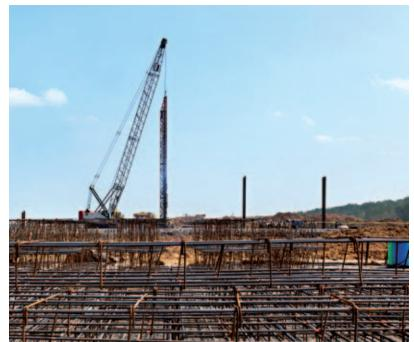
The wastewater pipes are in place. Now, it is time to lay the foundations for the production facilities and service buildings.
