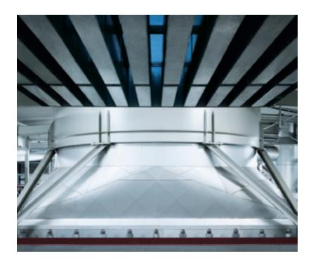
A heat-recovery steam generator above the gas turbine at Burghausen's modern CCGT power plant. Not only does the turbine meet a third of the site's electricity requirements, but its waste heat is used to generate process steam for chemical production. The superheated steam, in turn, drives other turbines to generate electricity. A perfect closed cycle that provides maximum efficiency, cuts costs and conserves resources.
