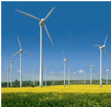
Enabling power plants
